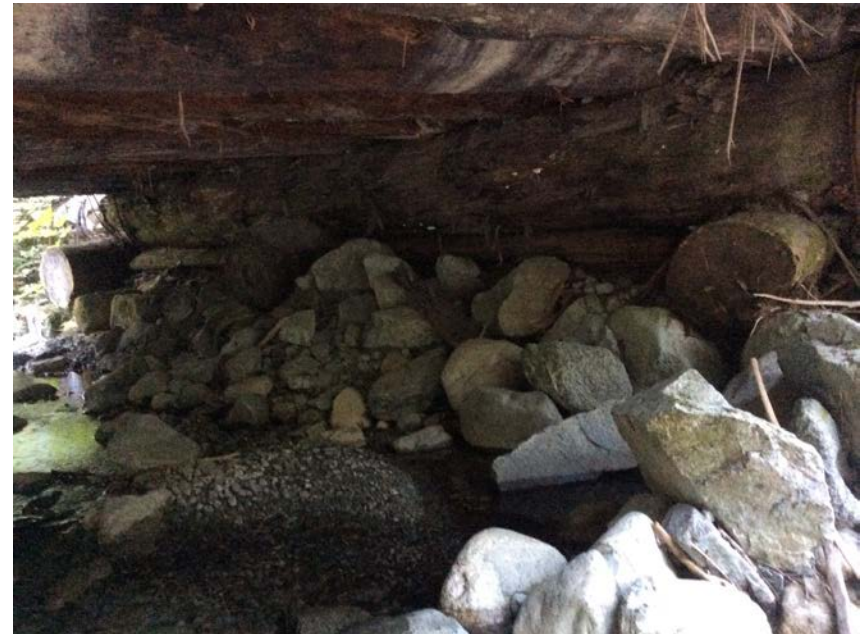
Right Bank Abutment when facing downstream
