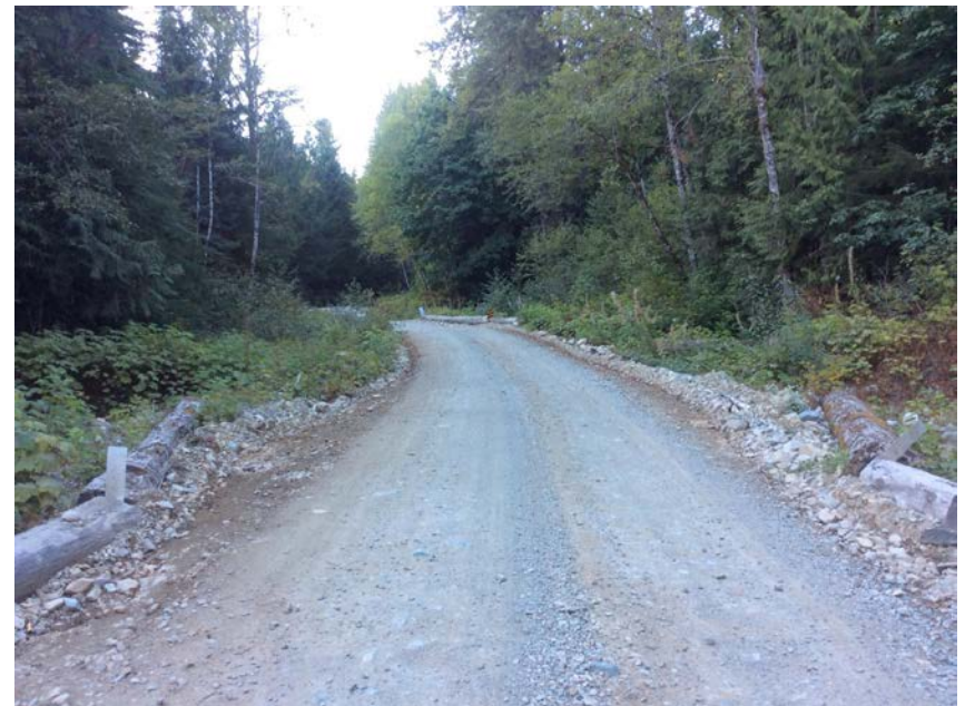
Right approach viewed from bridge
