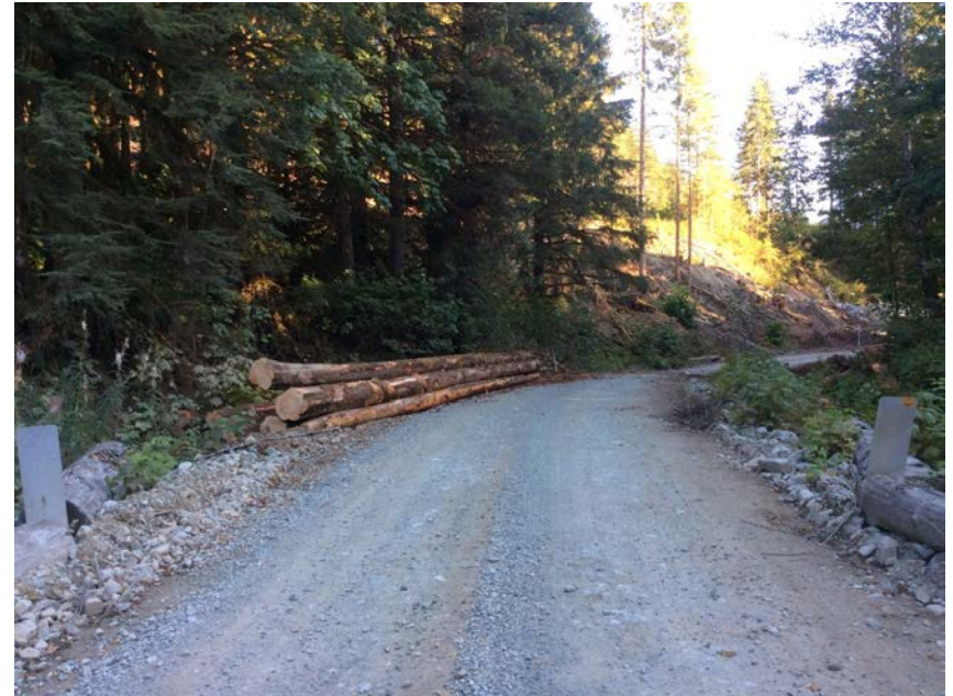
Left approach viewed from bridge
