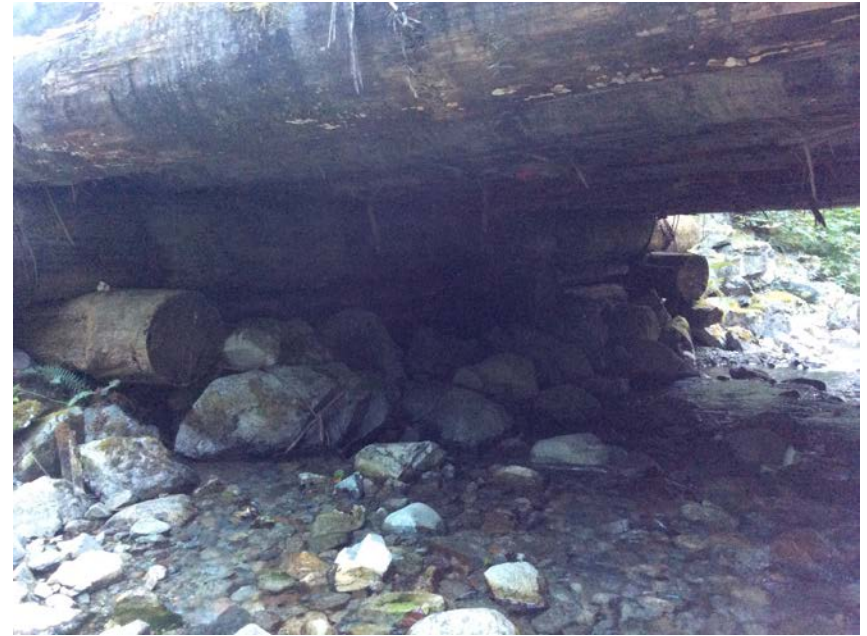
Left Bank Abutment when facing downstream
